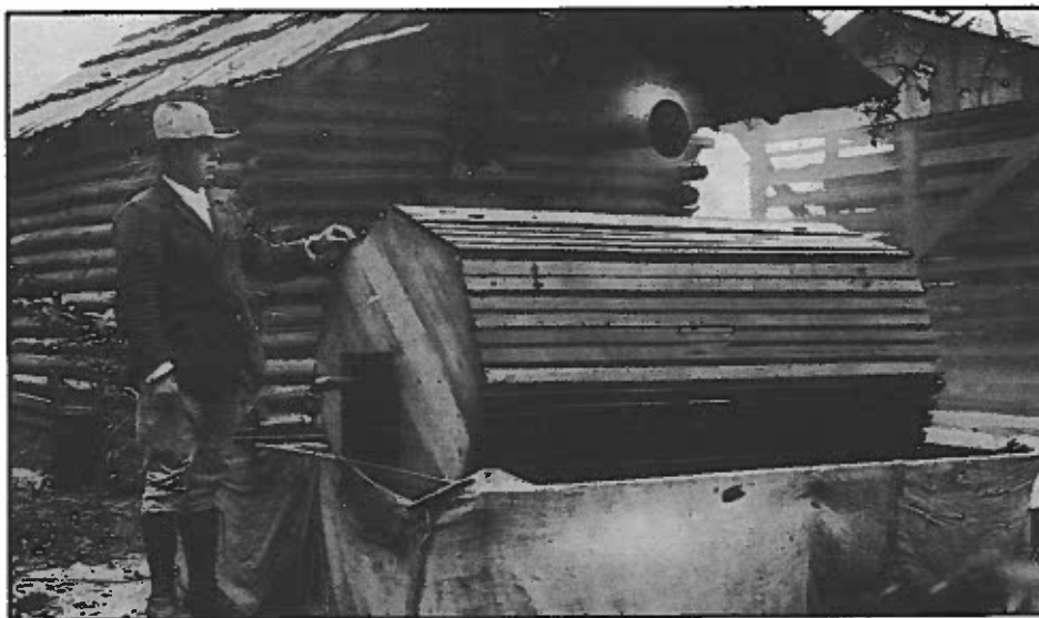
Charles Delaney in the 1920s is shown with a tumbler to extract seeds from cones dried in the log building.
